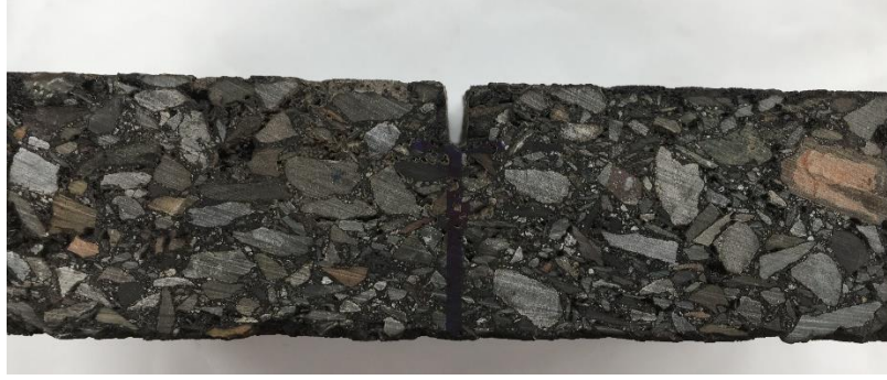
Figure 9. Notched asphalt sample.
